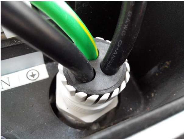
Picture 3 Use waterproof rubber sealing for wiring
