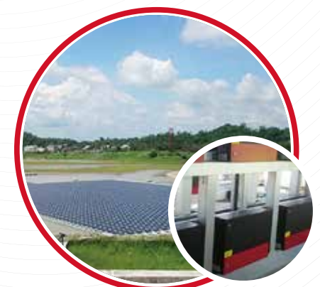
AGONG-DIAN RESERVOIR, KAOHSIUNG CITY, TAIWAN 2.3MW
